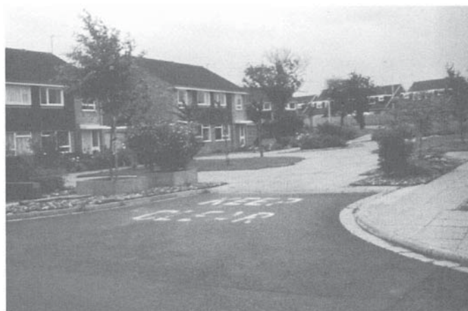
Fig. 26. British variation on the cul-de-sac , termed a “mixer court”; asphalt replaced by attractive paved court which permits auto-access and meets fire-safety regulations (Newcastle, U.K.).
